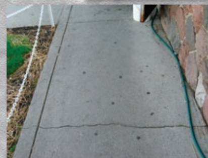
If you fail to properly design for shrinkage uncontrolled random cracks will occur
