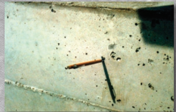
Bugholes on a plywood formed surface
