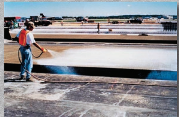
The proper application of a curing compound
