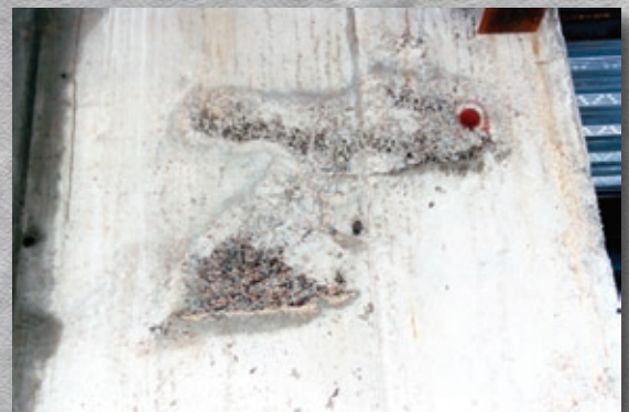
Honeycombing in a concrete column
