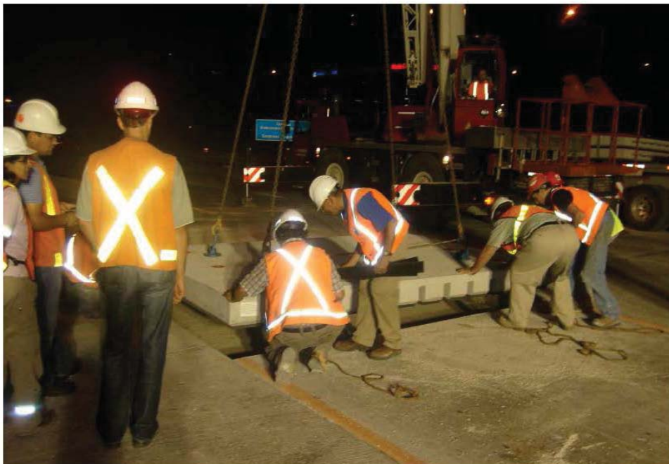
Figure 3.8 - Installation of Pre-cast Concrete Panel on Highway 427 (C/o super-slab.com).
