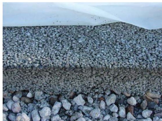
Figure 3.6 - Pervious concrete for a sidewalk application (provided by Concrete Ontario).
