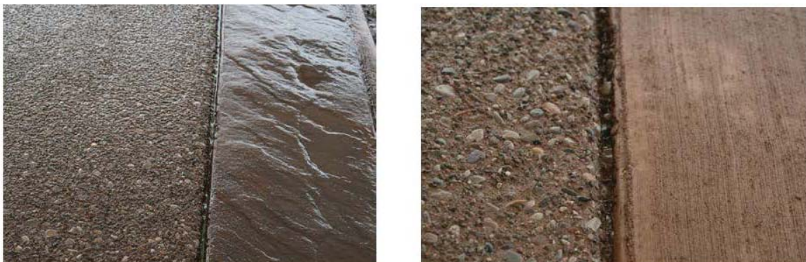
Figure 8.5 – Decorative coloured concrete with exposed, stamped and broom finishes (provided by Concrete Ontario).
