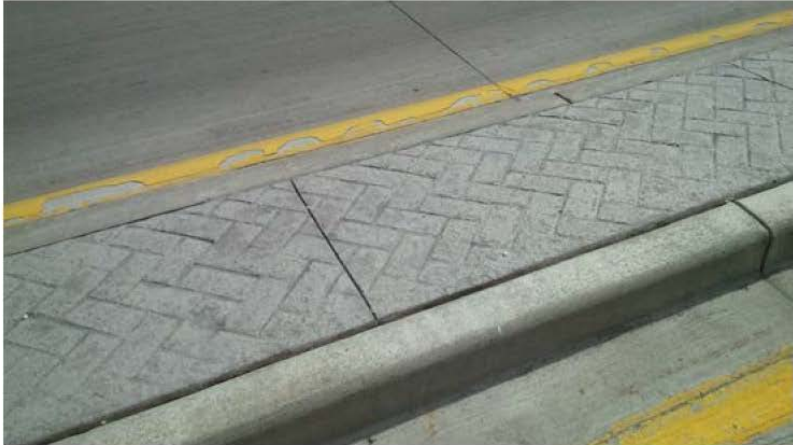
Figure 8.8 – Decorative coloured concrete with stamped stone finish (provided by Concrete Ontario)
