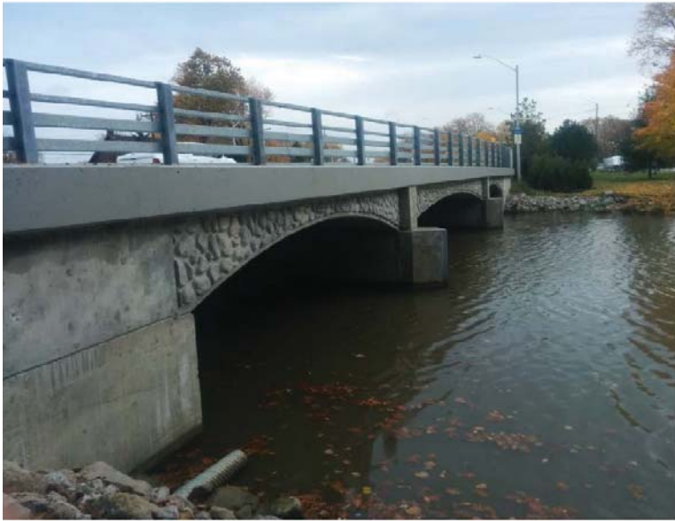
Figure 4.1 - Puce River Bridge at County Road 22, County of Essex
