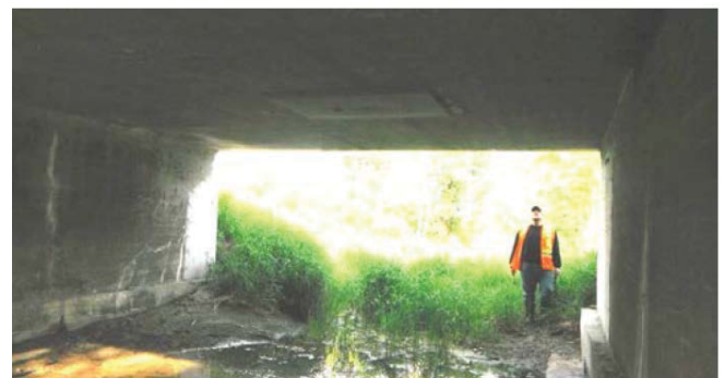
Figure 4.2 - Inspection of concrete frame bridge
