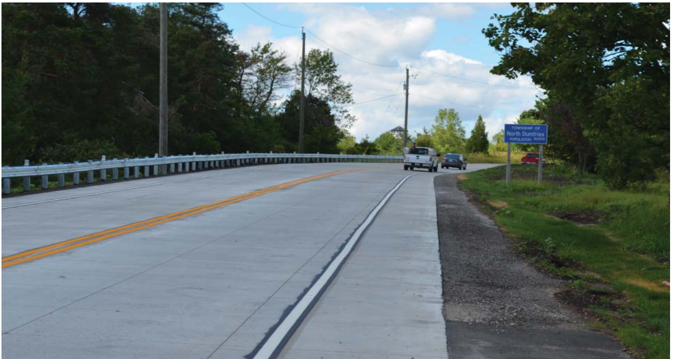
Figure 1.1 - Unbonded Concrete Overlay on Spragues Road (provided by Region of Waterloo)
