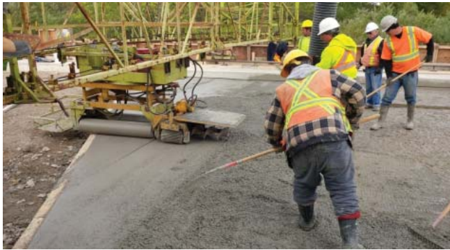
Figure 4.5 - Placement of concrete deck overlay 0
