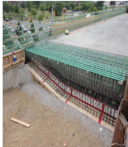
Figure 4.6 - Semi-integral joint and abutment retrofit
