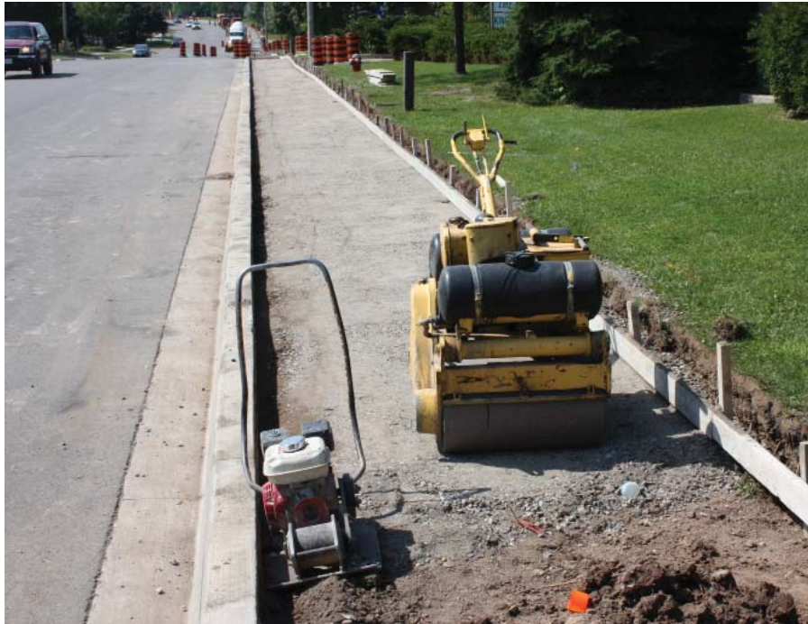
Figure 14.1: Concrete base and formwork preparation (provided by Mick Prieur)
