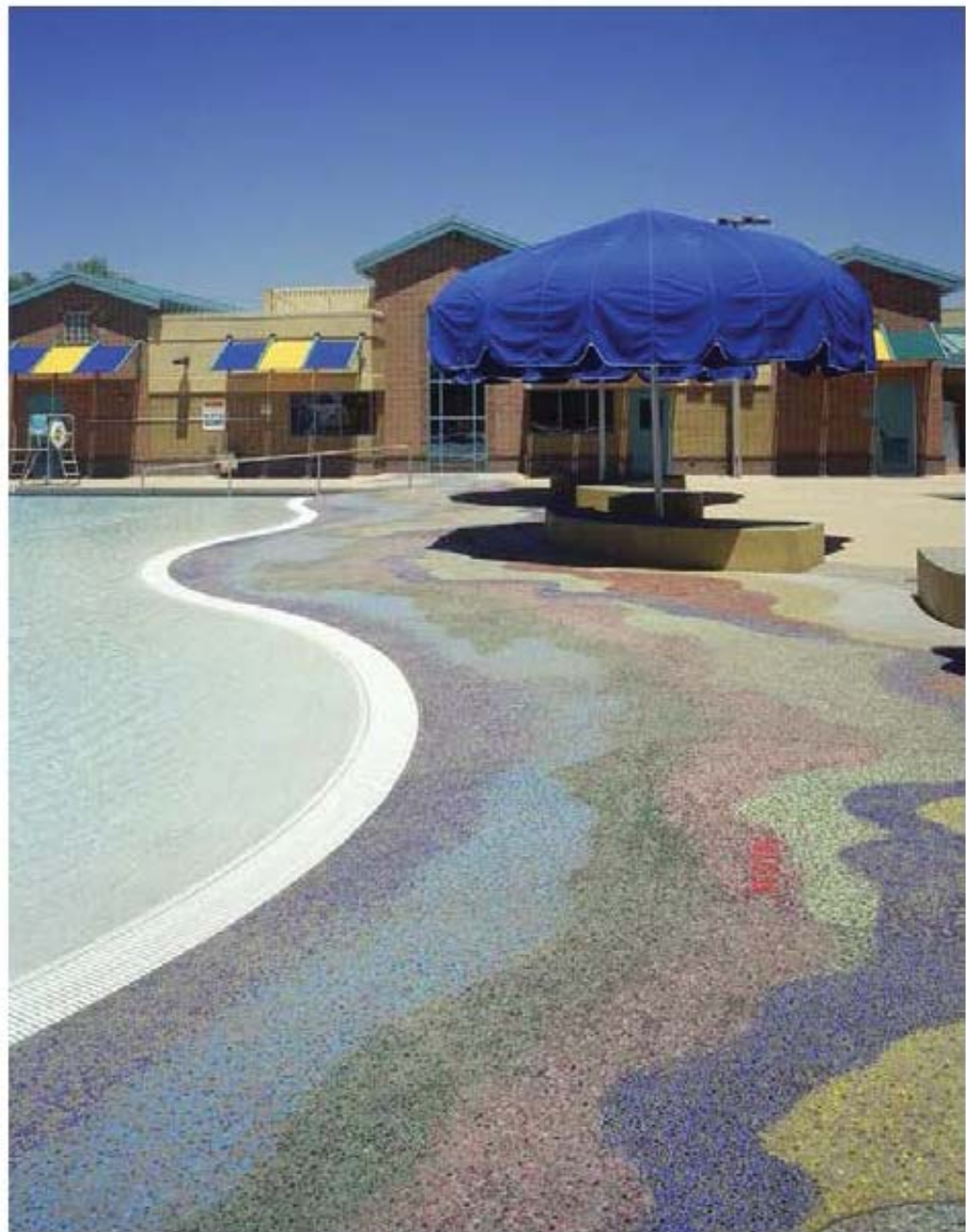
Figure 8.3 - Decorative patio and pool entry with exposed aggregate surface using coloured beaded glass (provided by Concrete Ontario)
