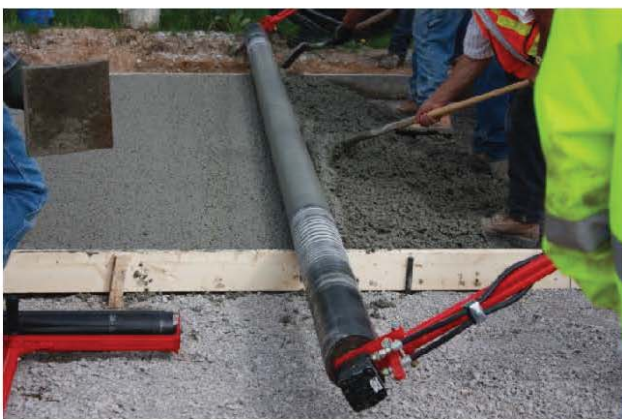
Figure 3.6 - Pervious concrete for a sidewalk application (provided by Concrete Ontario).
