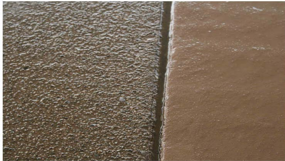
Figure 8.4 – Decorative coloured concrete with etched and stamped finishes (provided by Concrete Ontario).
