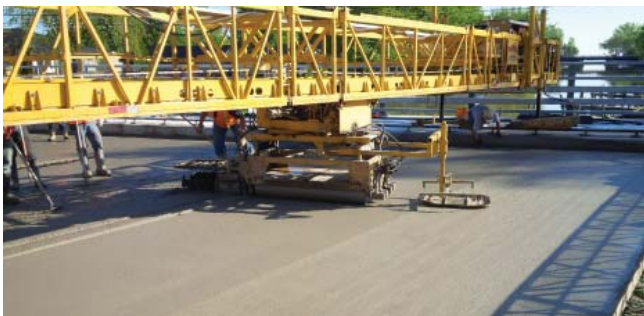
Figure 14.2: Concrete bridge deck (provided by County of Essex)
