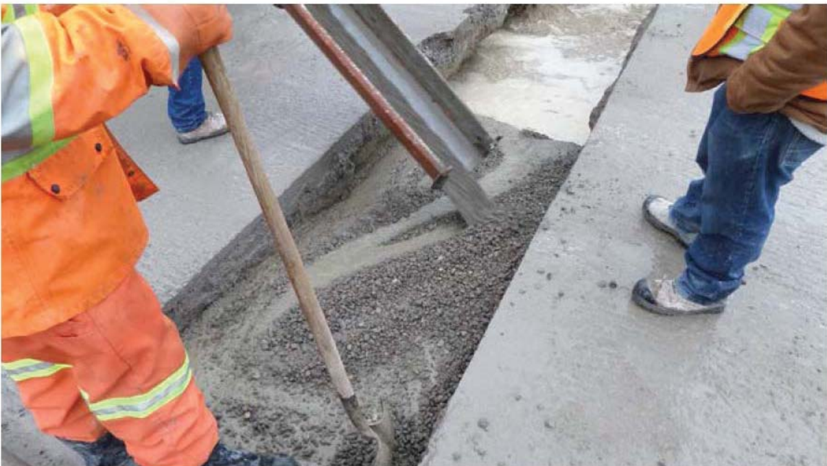
Figure 7.1 – Utility cut restoration with U-Fill (provided by CAC).
