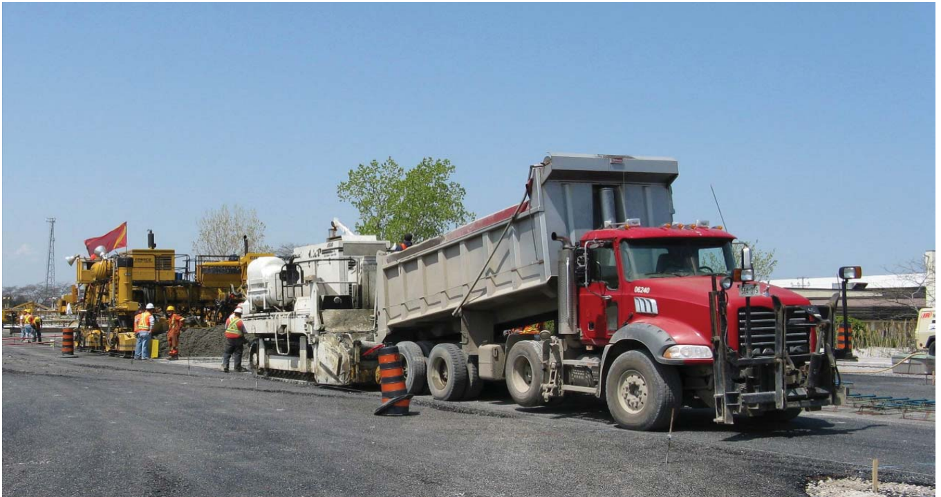
Figure 13.2: Concrete paving operation and dump truck (provided by County of Essex.)
