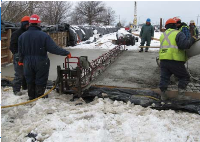
Figure 14.3: Vibratory screed concrete pour (provided by County of Essex)
